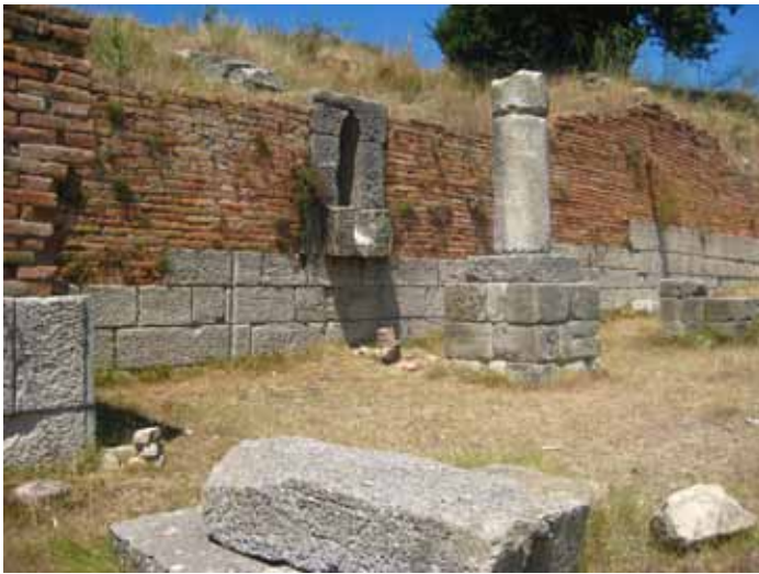
Fig. 24. Water outlet in Apollonia's city walls.
